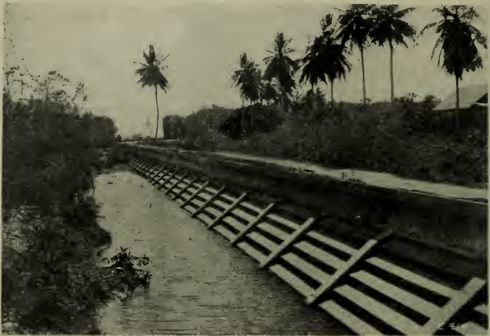
Fig. 5. Sea Wall at Rear of Tidal Marsh.
